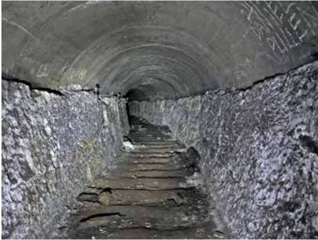
The Scenic Railway tunnel looking towards the Hereson Road terminus: note the restricted loading gauge. Photo Tim Wellburn
